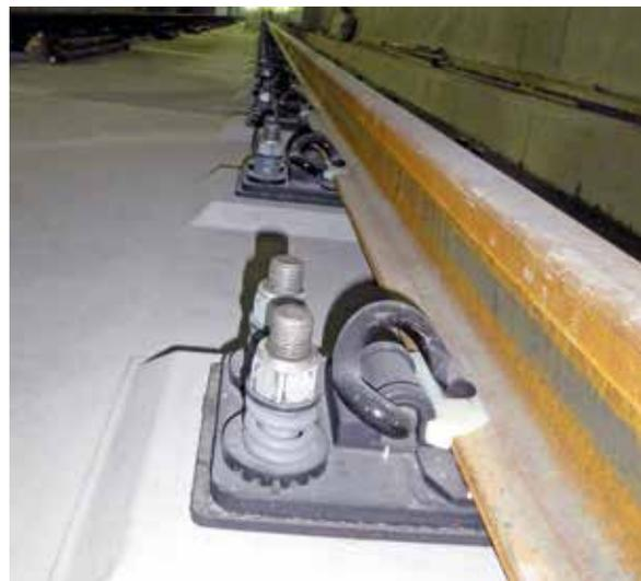
poured concrete plinth track due to the logistics involved in handling the large panels in the confined tunnel environment. Pandrol has continued to work closely with the trackworks contractor, Sampyo E&C, in order to optimise the construction method now being employed and the construction is now running smoothly.
